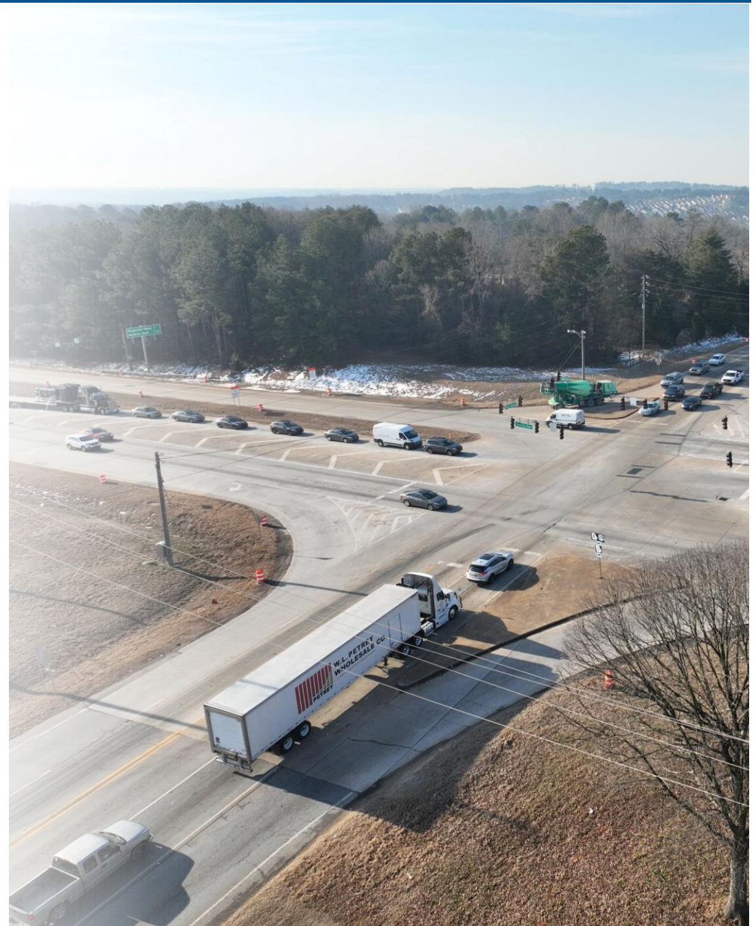
Photo of SR 316 at SR 8/US 29 Winder Highway
