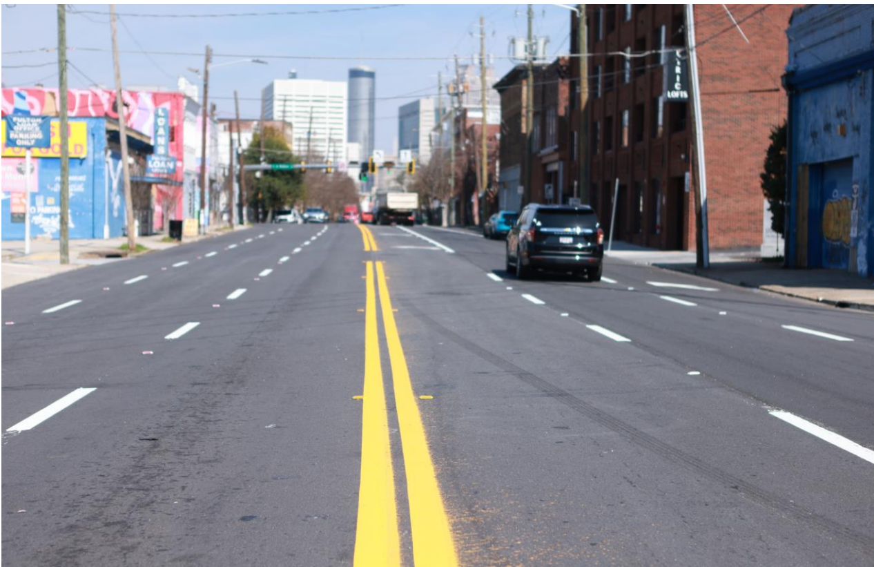
SR 14/Peters St at Hill Ave SE
