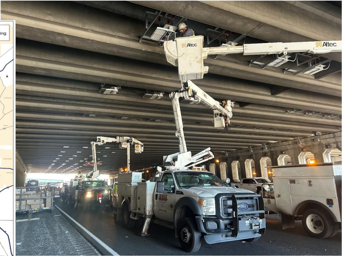
Tunnel Lighting Replacement I-75/85
